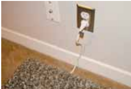
Hiding an extension cord under a rug can cause a fire.
