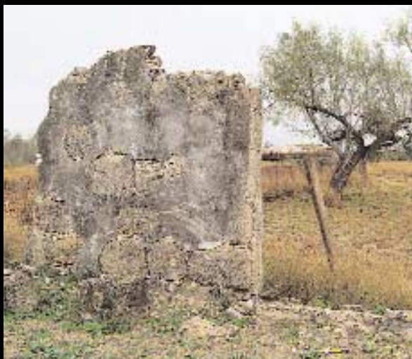
Left, a partial wall, the remains of Alfredo Villarreal's grandmother's house, shows the typical building method of South Texas ranchers of the late 1800s. Large blocks of caliche were stacked and cemented together with a mixture of lime and goat's milk, known as chipichil .
