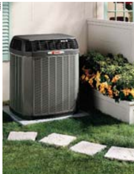
This is a two-stage outdoor heat pump unit installed at a home. It has a large condenser coil area for high efficiency.
