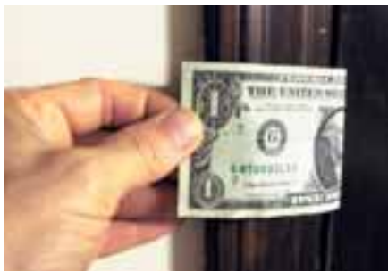
The dollar bill test is a quick and easy way to check the weatherstripping on doors.
