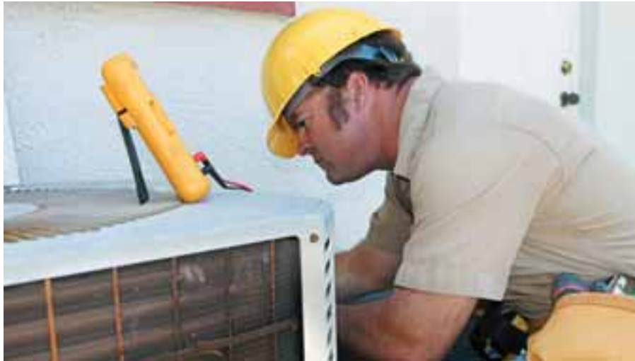
One of the best ways to save energy and extend the life of your air-conditioning system is to have it serviced annually by a qualified professional.
