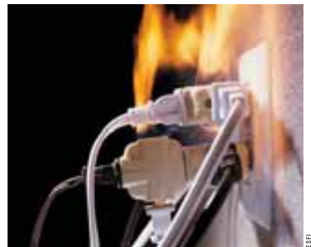
A power strip with over-current protection can help prevent fires.
