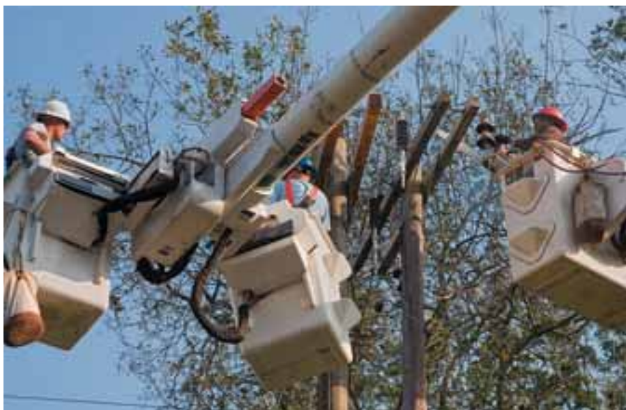
Construction crews work feverishly to replace damaged poles at Sam Houston EC.
