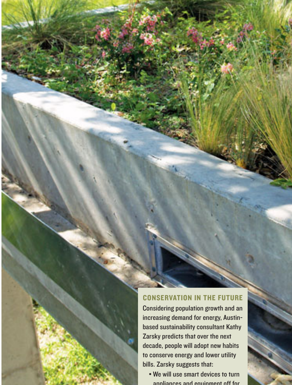
Detail of sod roof edge and gutter
