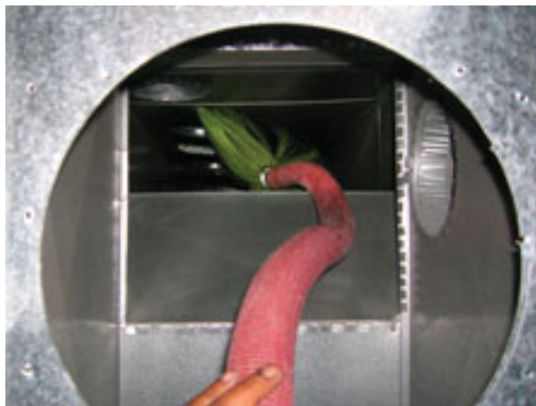
This duct is being cleaned with an air whip and vacuum unit. Joints and protrusions are likely places for dirt to collect in a duct.
