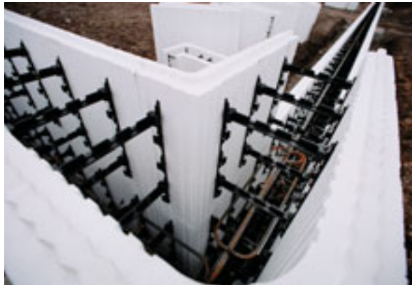
These insulated concrete forms use webs between the foam panels to create the width of the gap for the concrete.
