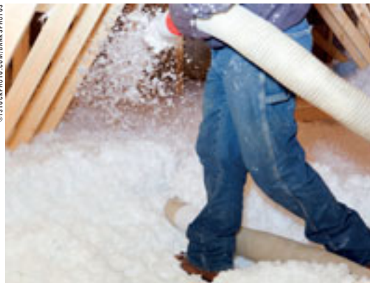
Nope, it's not snowing. It's loose-fill insulation being blown in—one of many insulation choices.
