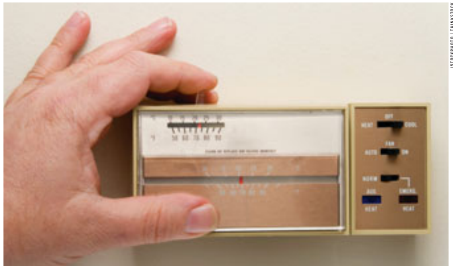
Setting back your thermostat in the winter can save energy and money. And, if your thermostat looks like this one, there are even more savings awaiting you by replacing it with a programmable version.
