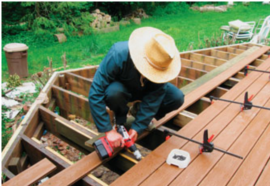
Using clamps when installing decking helps ensure perfect plank spacing.
