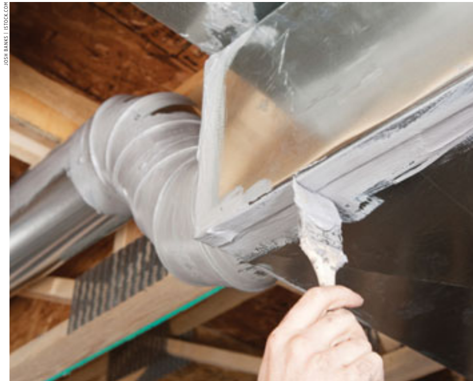
Need to seal your ducts? Don't reach for the duct tape. Use a mastic sealant or metal tape.
